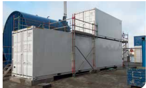
Completed land demonstrator in Kiel
