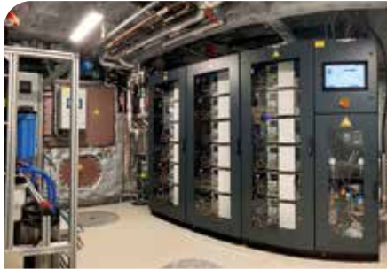
Fuel cell cabinet of the demonstrator
